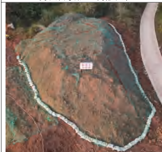
龙凤寺隧洞出口表土堆放及防护
